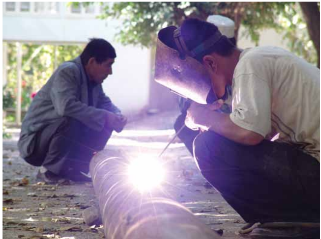
Community members contribute their labour to a local public works project.
